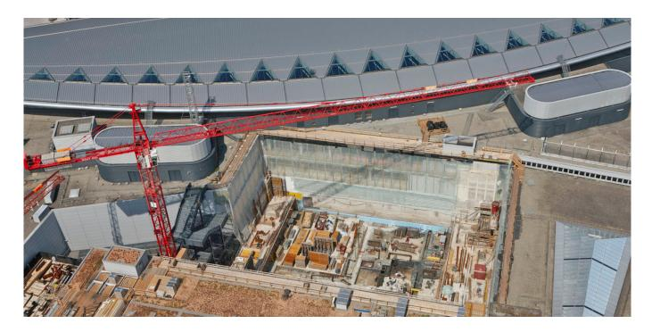
In the middle of Zurich Airport, a modern, central security control building is being built. In close cooperation with the project manager, EBP are planning a structural framework designed to take current and future security aspects into account
