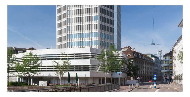
EBP originally inspected the earthquake resistance of the Zurich high-rise's (Hochhaus zur Schanzenbrücke) load-bearing structure in 2006. We again carried out a similar inspection in 2020, while also completing a general evaluation of the load-bearing structure (e.g. punching shear, fire protection, watertightness) and the conditions that would have to be met for any major structural changes (including additional stories and replacement).
