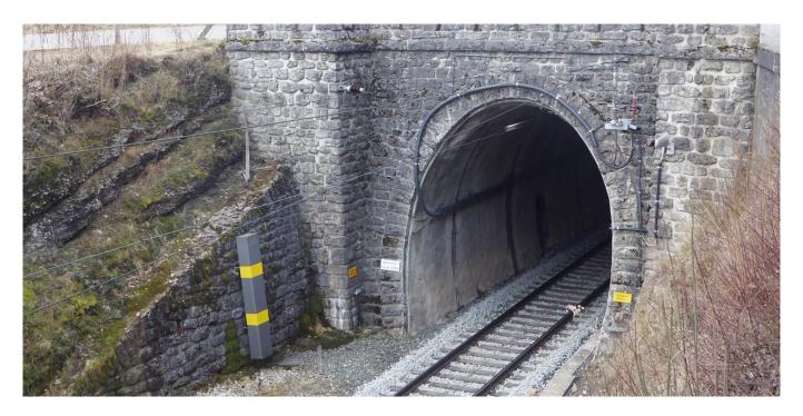
As part of the renovation of the Wasserfluh Tunnel (2<sup>nd</sup> stage), the existing single-track railway tunnel (length 3,556 m) had to be repaired and equipped with a ballastless track. EBP was responsible for the comparison of various options for the construction of the track and for the speed optimization as well as for producing the preliminary project from the best option.
