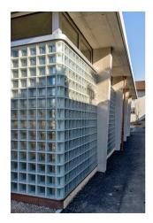
The same basic architectural design was used for the gymnasium. One exception, however, was the gymnasium's large prefab glass-brick walls that are supported by the concrete elements and attached laterally to the columns. Skylight ribbon-window frames made of metal are mounted above the glass-brick walls. Some of the win-dows themselves can be opened.
