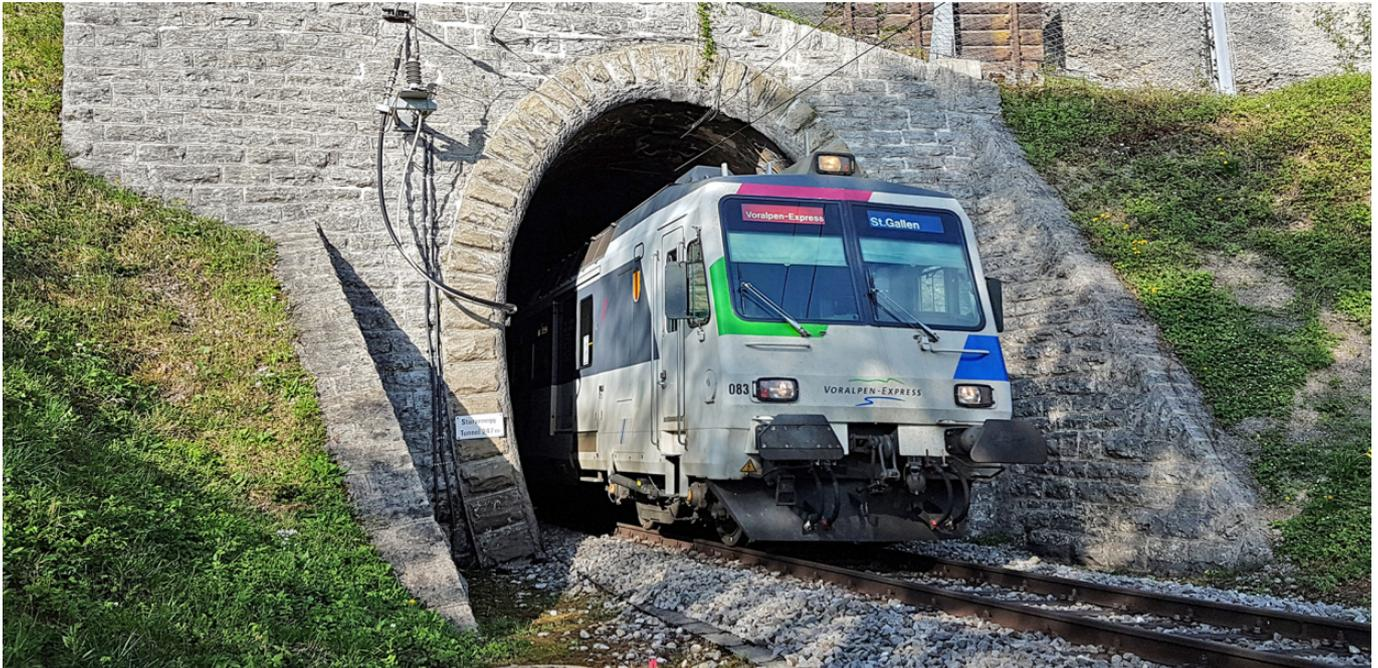
**Swiss Southeastern Railway has commissioned EBP to complete the planning for the necessary renovation of the Sturzenegg Tunnel, which was originally built in 1910. The aim of the renovation measures is to guarantee compliance with the applicable structure-gauge requirements and to secure the tunnel's serviceability and long-term structural integrity. The scope of EBP's work also includes issuing invitations to tender and managing the project's realization.**
