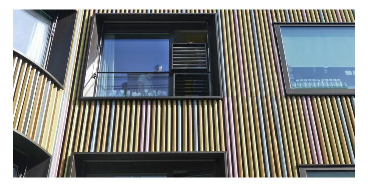
After the newly built daycare center at ETH Zurich opened its doors to its children, the building's passive air-conditioning system failed to function properly, as evidenced by overheating in the spring and summer. The reasons for the overheating proved to be complex. After analyzing the situation, EBP proposed a suitable solution, completed the corresponding planning work and oversaw the corrective measures.
