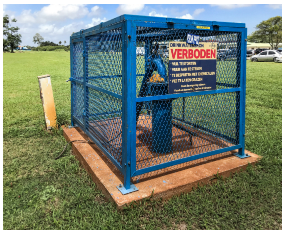
Paramaribo area, Suriname: Protected groundwater well
