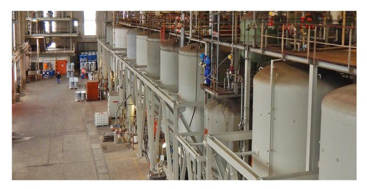
EBP was commissioned by CABB AG to carry out seismicsafety analyses of its steel tanks for hazardous materials, as well as to plan the implementation of any necessary seismicretrofitting measures in a manner that would not force the company to interrupt its operations.
