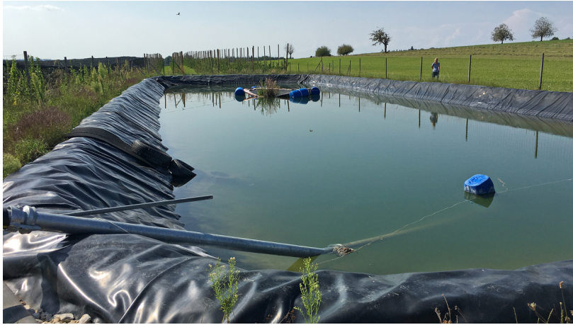
Pond with geomembrane liner, drainage pipe, and tire ladder
