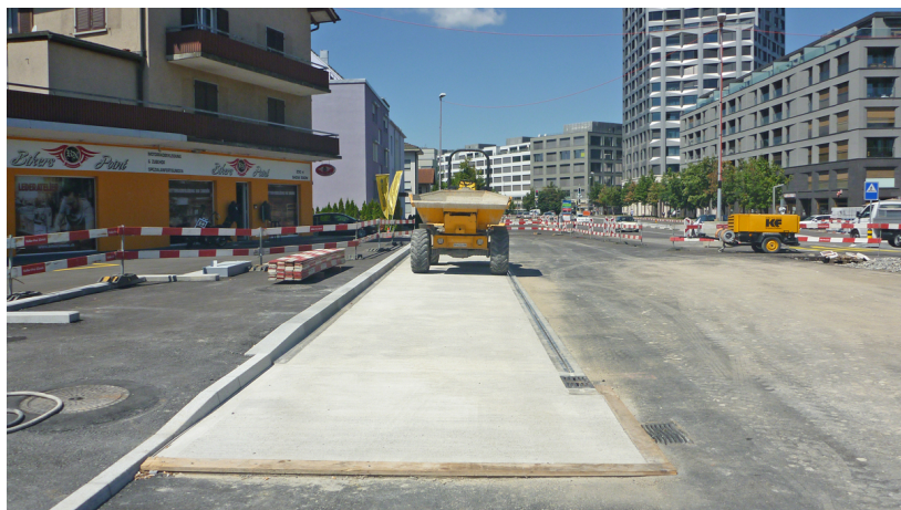
Bus stop with slot drainage along the edge of the asphalt: Securro Slimline
