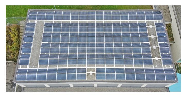
In the course of an energy renovation, the "Chappelistein" primary school building in Ottenbach received a new photovoltaic system on the roof of the gymnasium. We took on the technical planning and implementation support for the photovoltaic system as well as the replacement of the thermal systems. The Ottenbach primary school is now equipped with a photovoltaic system with an output power of around 55 kWp and an annual solar-energy yield of around 50 MWh.
