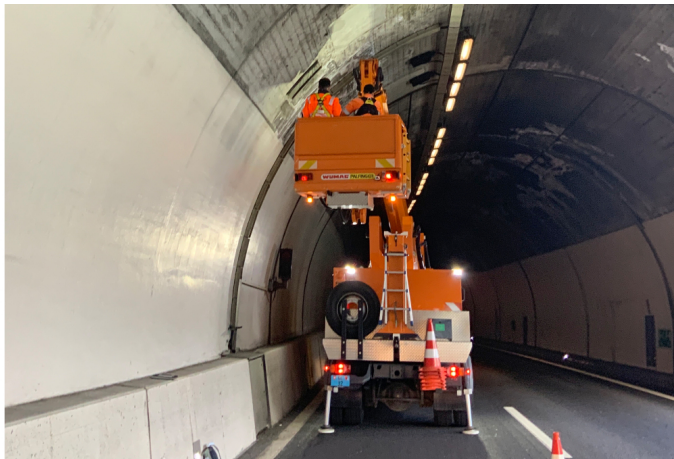
Tunnel condition inspection
