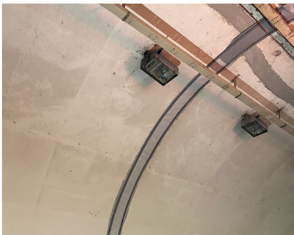
Site management waterproofing block joints
