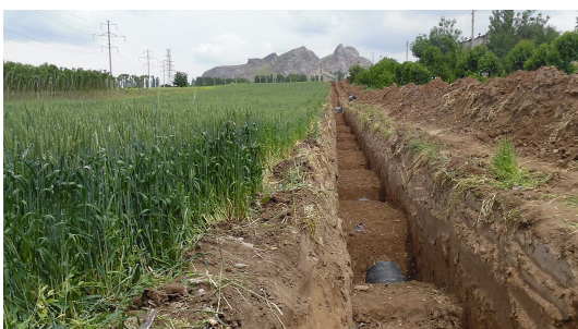
Renovation of drinking water and wastewater infrastructure in Osh and Jalal-Abad, sewerage in Osh, Kyrgyzstan
