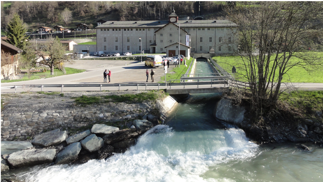
Underwater canal at the Küblis Power Plant
