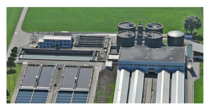
The Glarnerland Wastewater Treatment Association (AVG) plans to rehabilitate the wastewater treatment plant (WWTP) Glarnerland, to extend its capacity from 70'000 to 105'000 Person Equivalents (PE) and to implement advanced treatment for the elimina-tion of micropollutants. EBP supports AVG with the procurement of the design and implementation consultancy.
