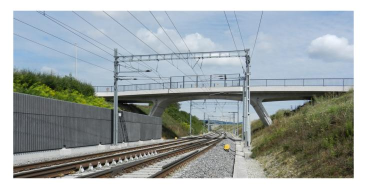
Given that it had become a bottleneck, the Swiss Federal Railways (SBB) rail line between Hüntwangen and Neuhausen was expanded from a single-track line to a double-track line. EBP played a leading role in the project's planning and realization.
